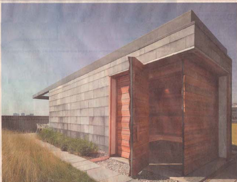
The rooftop sauna at Kenneth Montague's west end Toronto condo camouflages a homely elevator housing. BEN KAPPA/FRAME
